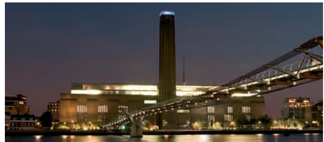
Tate Modern and National Portrait Gallery, London Equation Lighting Design, Advanced Lighting Technology
